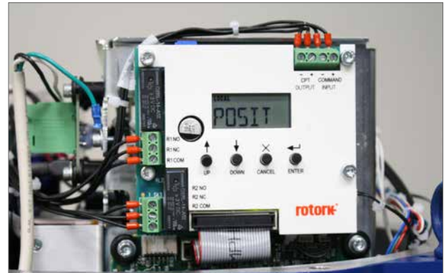
Fig 6.32 Control input connection
