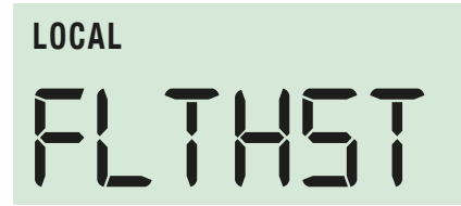
Fig 8.1 Fault history menu
