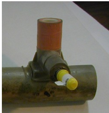
ALDYL-A TEE AFTER SCRAPING
