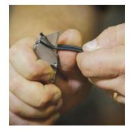
Score down the shield and completely separate wires encapsulated in the semi conductor.
