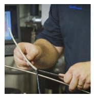
Score heat trace insulation jacket down the center to the end. Peel off insulation.
