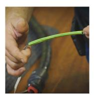
Prepare the ground. Insert the braided ground into the green/yellow striped ground braid protector sleeve. Insert end into a spade lug and clamp to secure.
