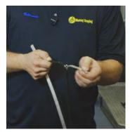
Score heat trace 6" from the end. Bend as needed to expose wires.
